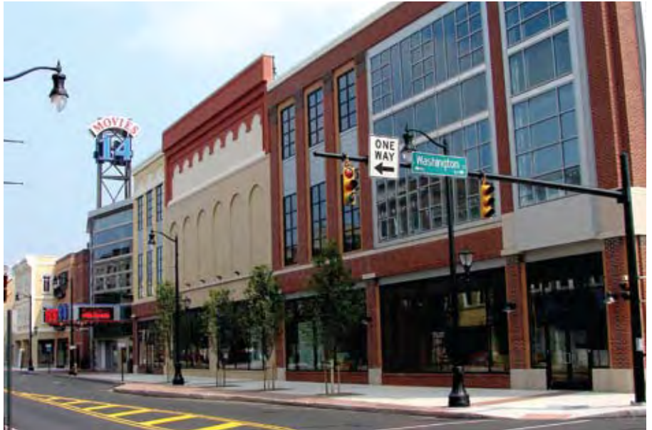
University Corners is an approximately 120,000-square-foot mixed-use development in downtown Wilkes-Barre, Pennsylvania.
